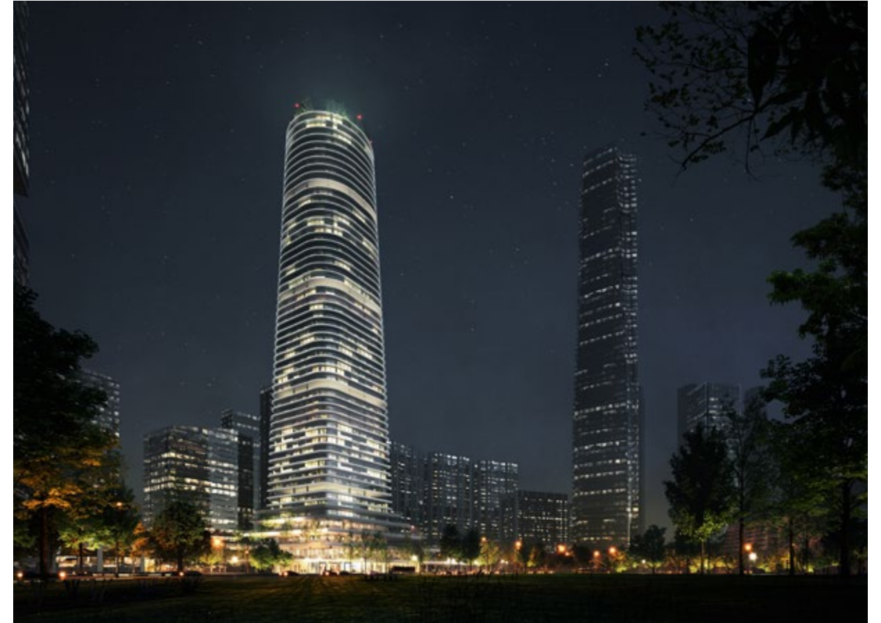
Exterior view towards Southwest (nighttime)
