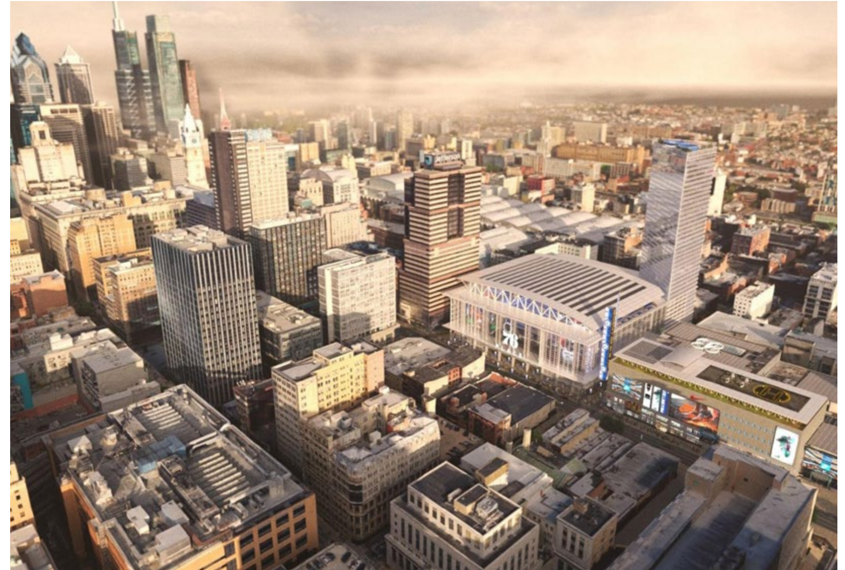
Exterior aerial at Market Street
