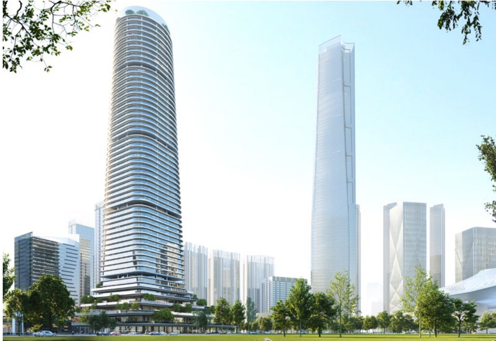
Exterior view towards Southwest (daytime)
